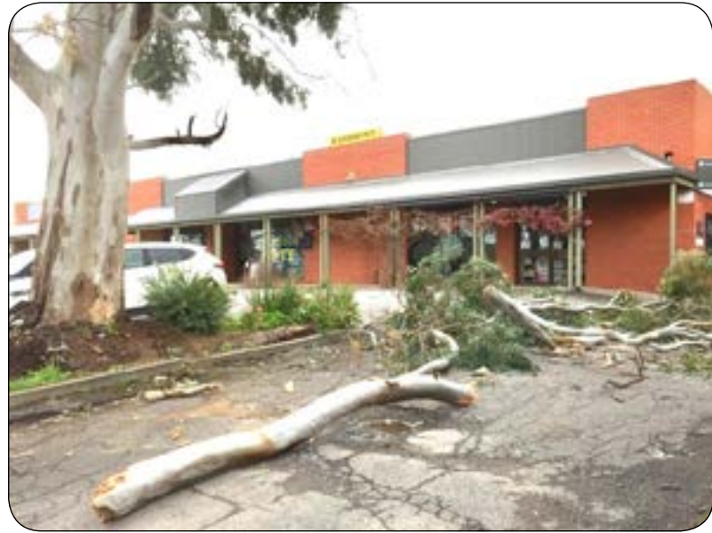
◆ Photo - Trees are essential for our survival, but why would you plant a shrub, that has the potential to grow into a 6 metre tree, in a car park zone? And it is guaranteed, that at some stage, it will shed or drop branches at times of stress. Fortunately, no one was injured when a large limb from this tree broke off and crashed to the ground.
